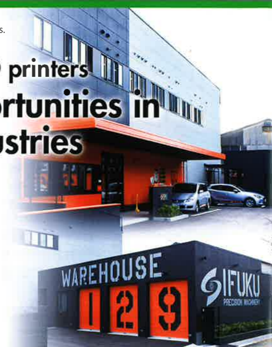
The new head plant completed in August 2017
